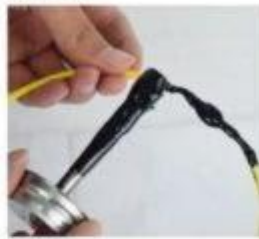
2. Apply liquid tape to wire
